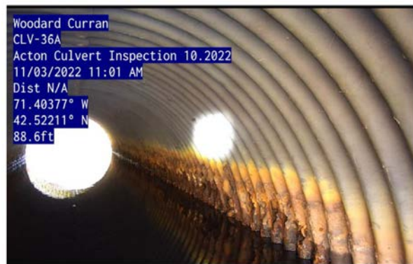
Photo 3-1: CLV-36A – Zoom camera video snapshot showing deterioration in a culvert
