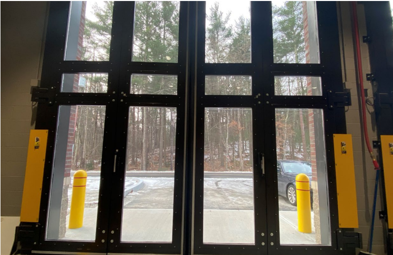
Bifold door installation
