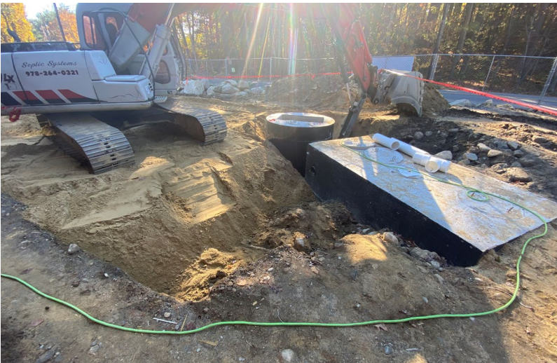
Septic system installation
