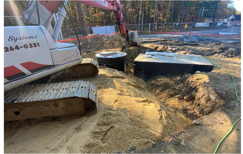
Septic system installation
