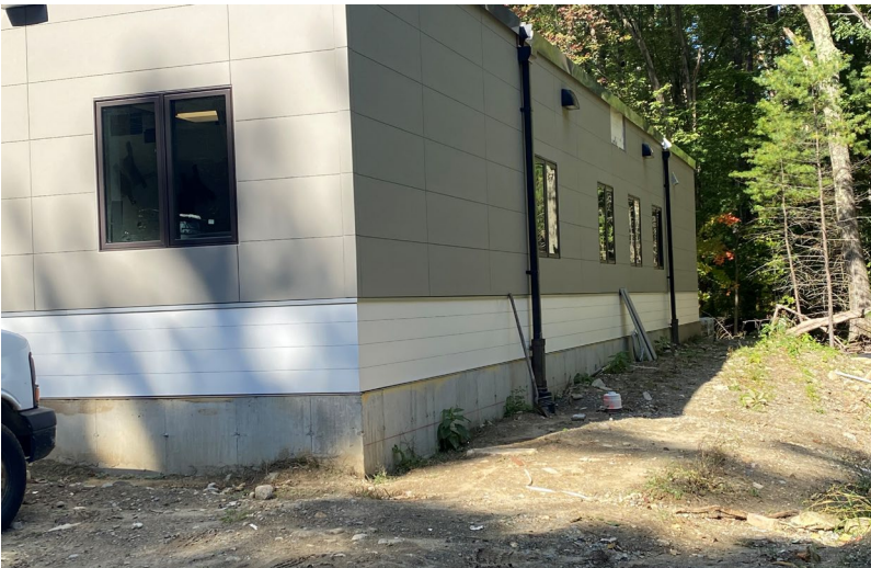
Down spouts installed around the building
