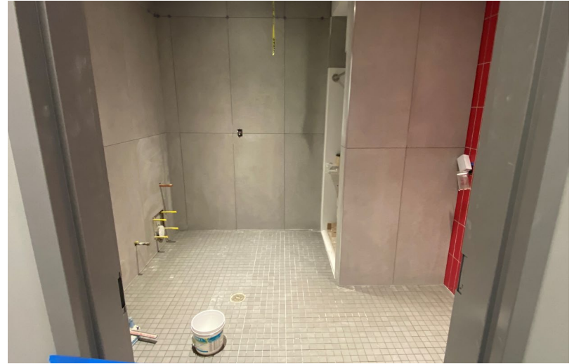
Ceramic tile installation in bathroom
