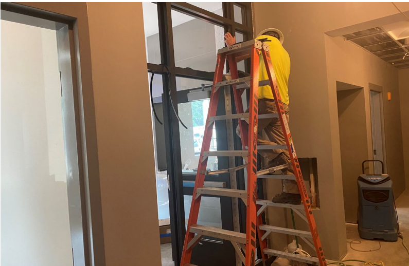
Installing front door glass
