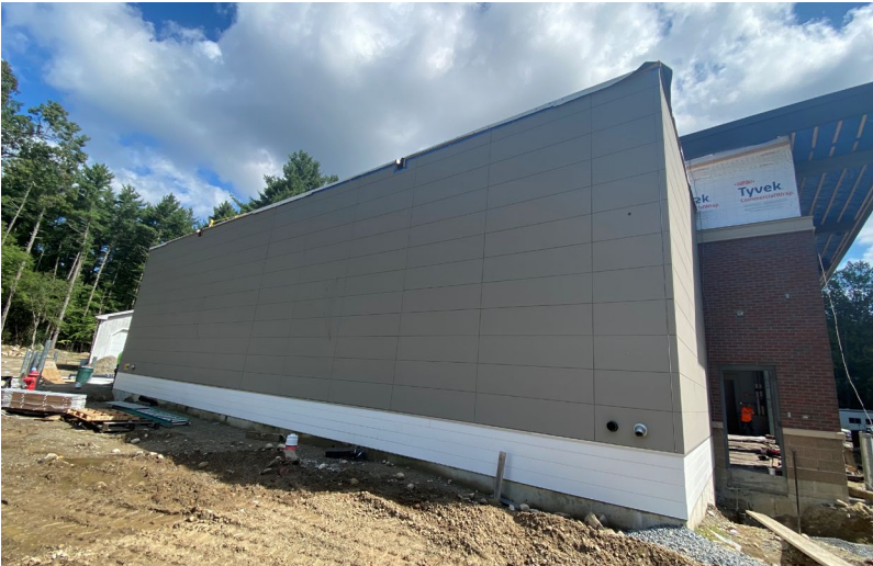
Complete Nichiha siding of the west side of building
