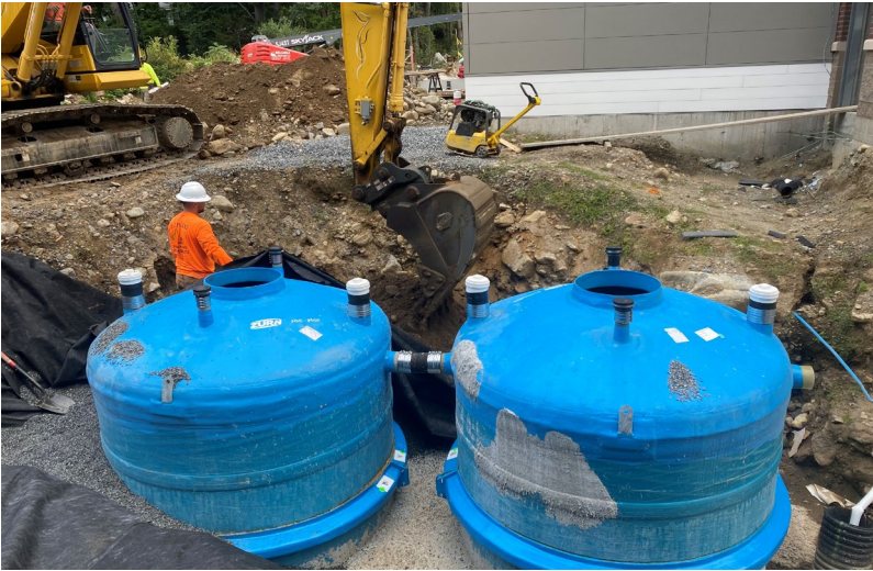
GSI tank backfilling
