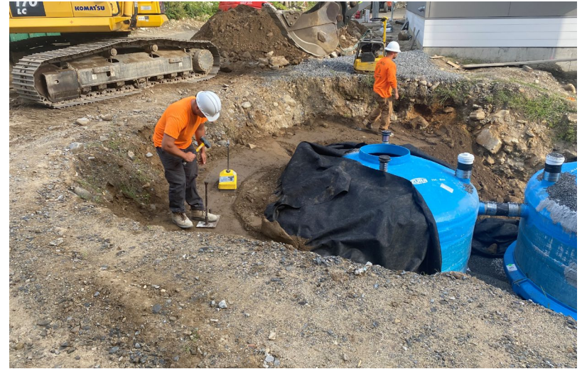
Atane onsite performing test soils
