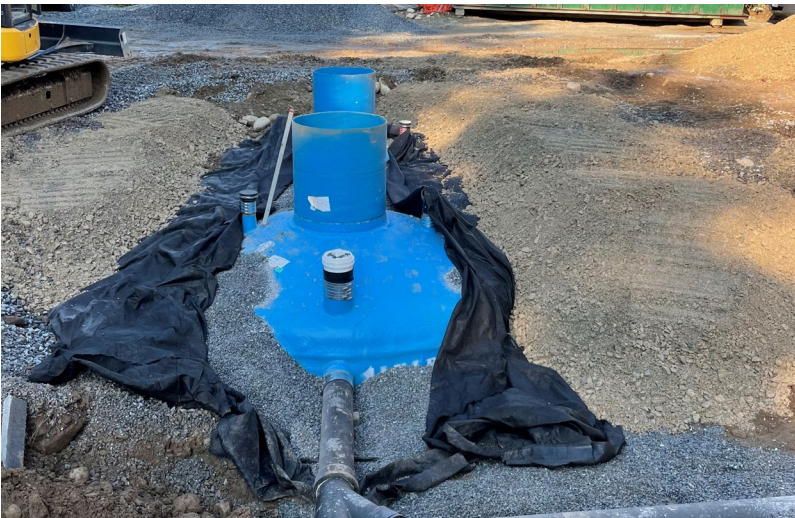
Vent has been installed
