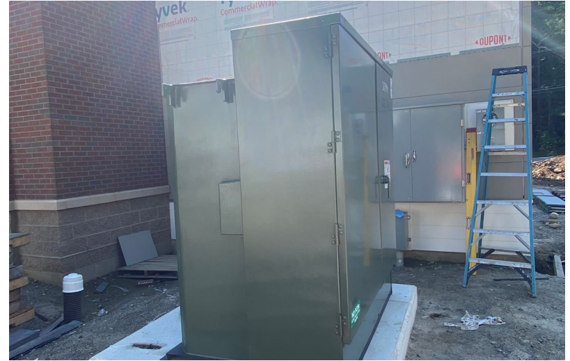
Transformer has been installed
