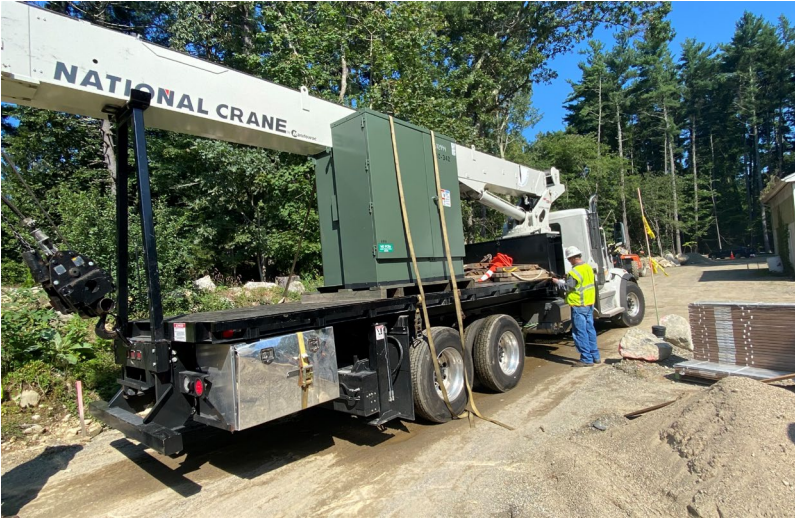
Eversource deliver the transformer
