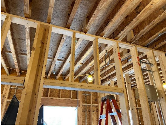
HVAC hangers installed on east side (03/05/2021)
