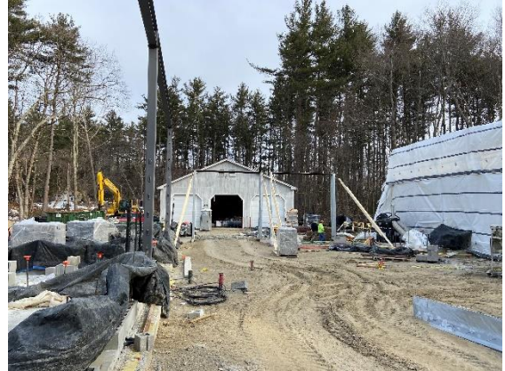
CMU frames erected on north side of apparatus bay (03/05/2021)
