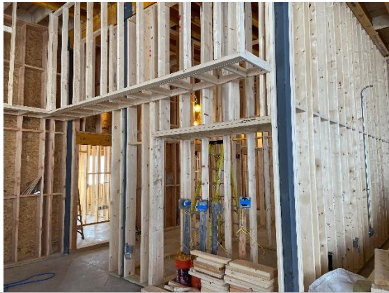
Interior soffit installation (02/10/2021)
