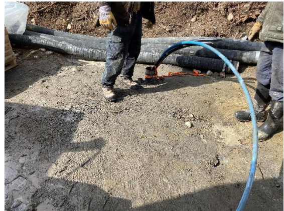
Grouting operations at geothermal wells (03/04/2021)
