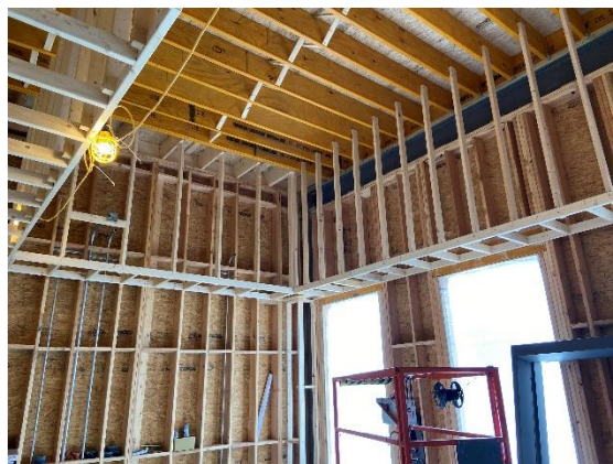
Interior soffit and time capsule box out installation (02/23/2021)
