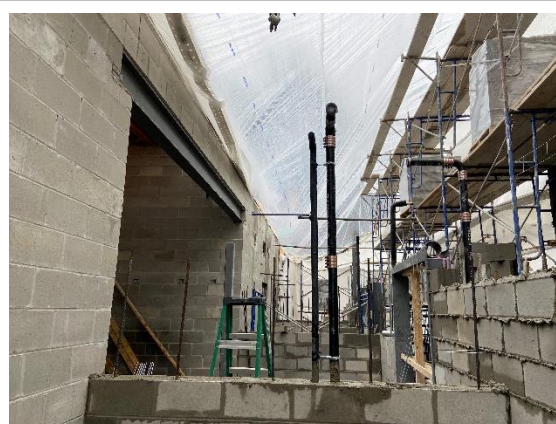
Masonry construction and rough-ins between Line 5 and 6 (03/01/2021)
