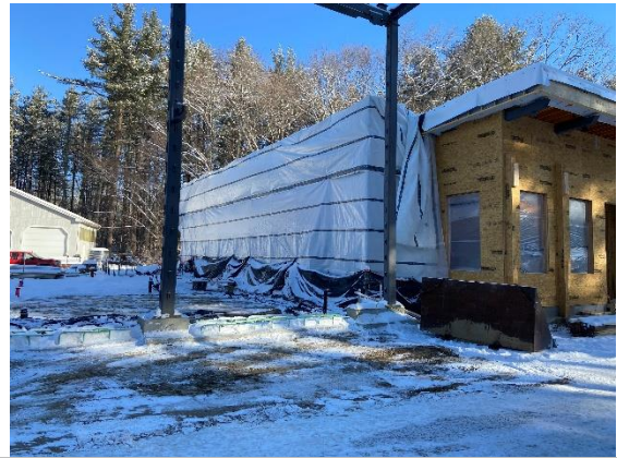
Enclosure for masonry construction (02/10/2021)
