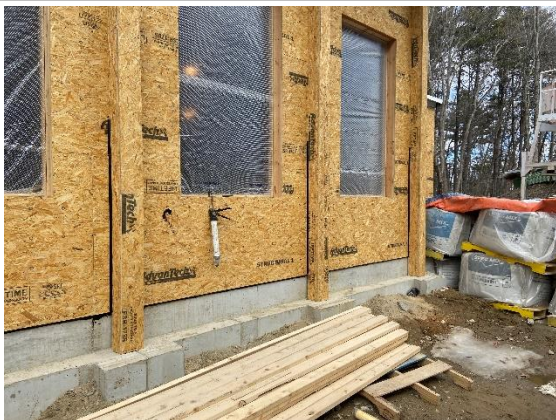
Waterproofing installation on southeast face (03/04/2021)
