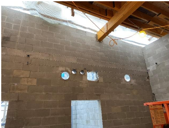
LVL bearing connection at masonry wall at Line 6.5 (03/04/2021)
