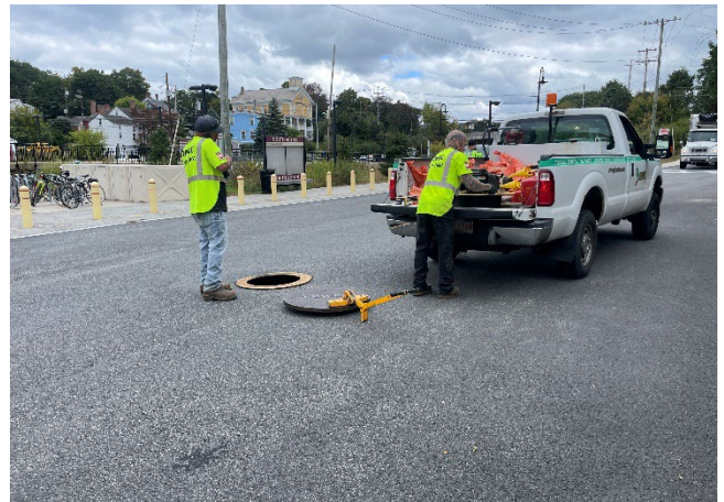
Above: Contracted crews completing smoke testing to identify areas in the sewer system where there might be inflow and infiltration (I/I).
