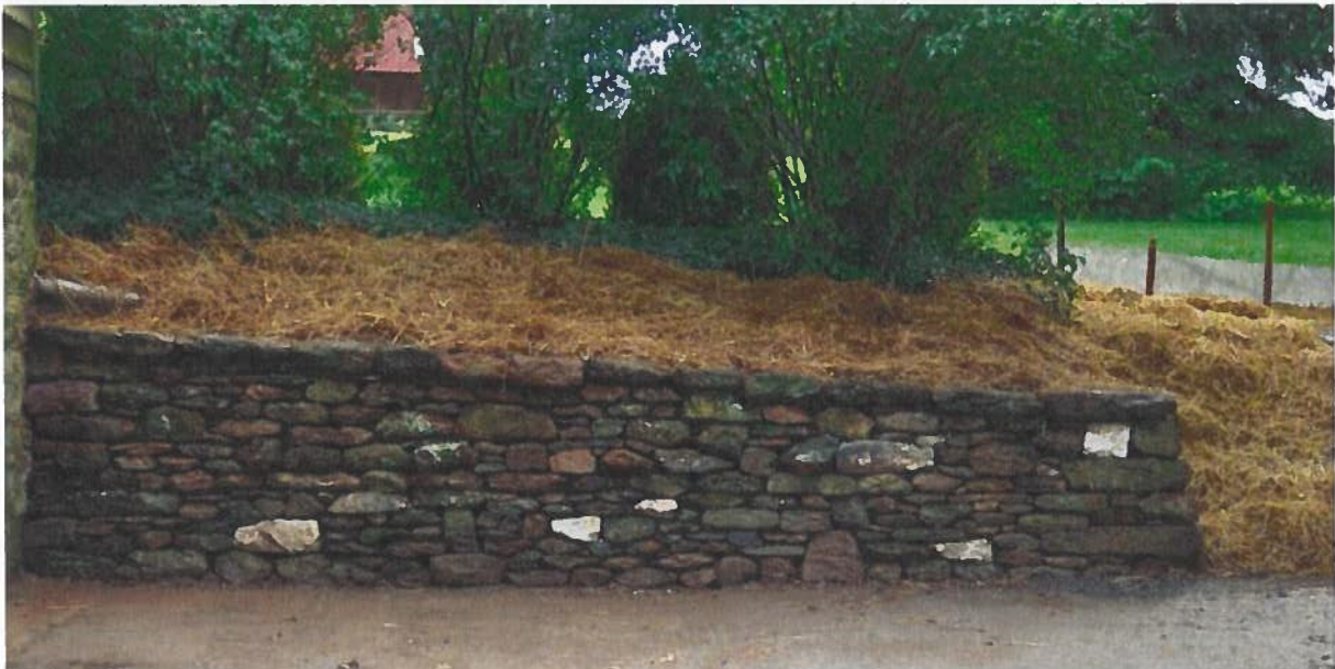
Below: New England's typical dry set natural stone wall, with larger top row as a cap to stop water.
